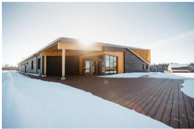
Cultural Gathering Centre, Métis Crossing, designed by Métis Architect Tiffany Shaw-Collinge. Photo courtesy of the Métis Crossing website: https://metiscrossing.com/cultural-gatherings/
